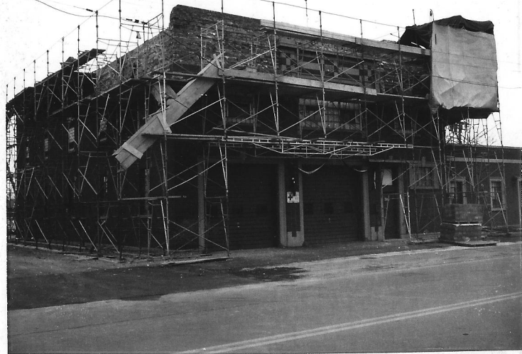
Progress on November 16, 1966 Front Elevation
